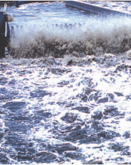
Brush Aerators in an Oxidation Ditch
